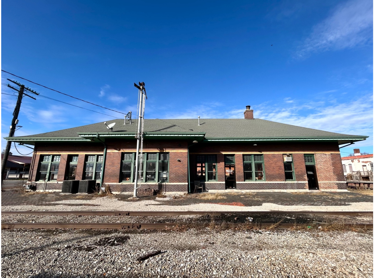
Figure 10: Facing northwest toward the southeast elevation of the Burlington & Wabash Railroad Passenger Depot at 1 Elm Street (LS-AS-003-0046; Parcel 11-01.00-01-2-30-08.00).
