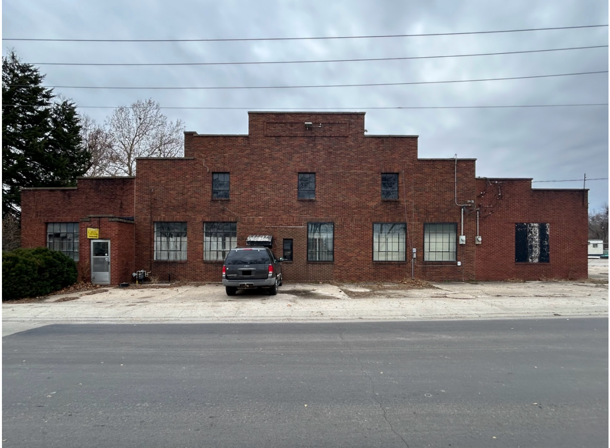
Figure 20: Facing west toward the primary east façade of the 1910 brick warehouse located at 10 Hickory Street (LS-AS-003-0062; Parcel 11-01.00-01-2-23-08.00).
