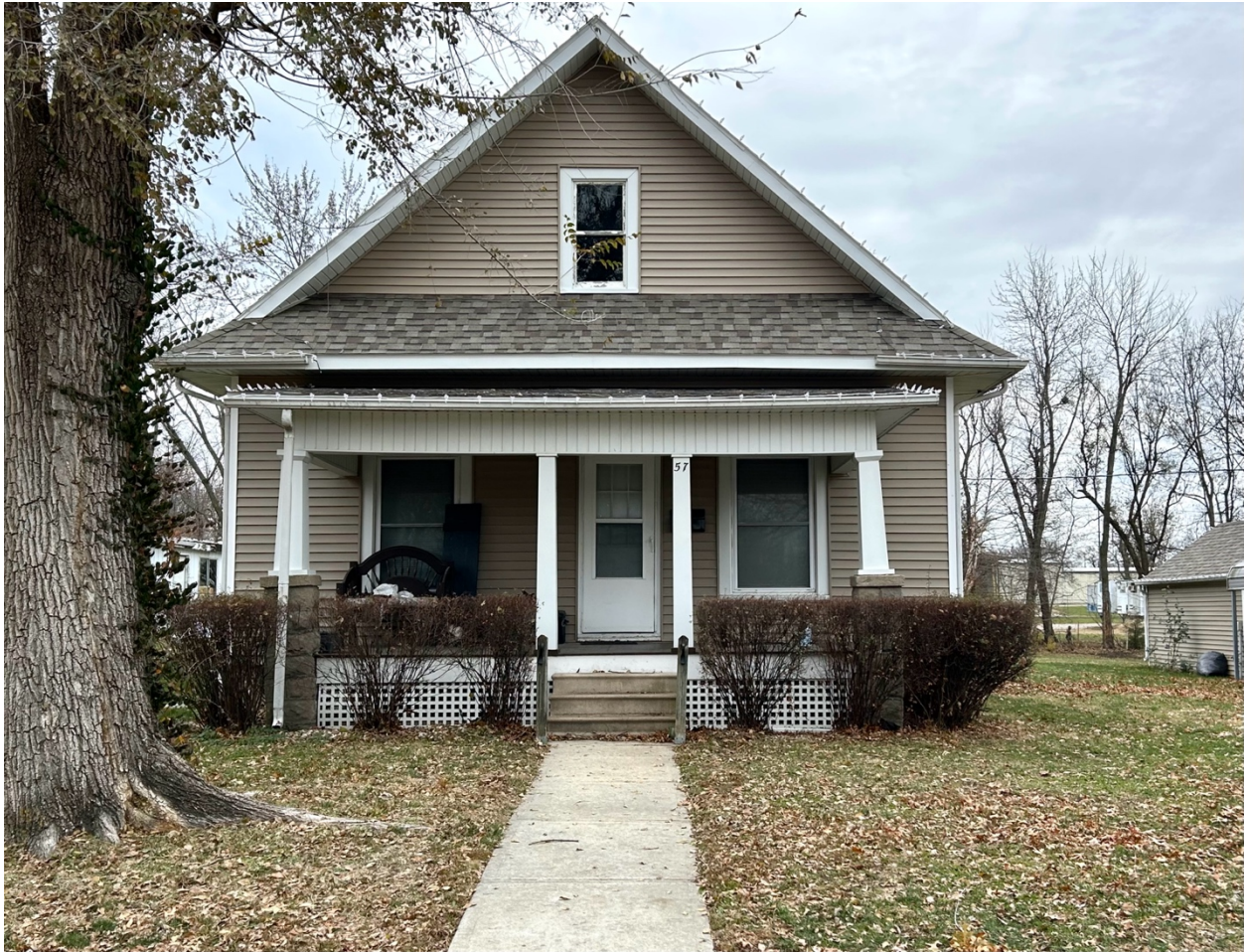
Figure 12: Facing east toward the west elevation of the dwelling located at 57 Wilson Street (LS-AS-003-0117; Parcel 11-01.00-01-2-23-06.00).
