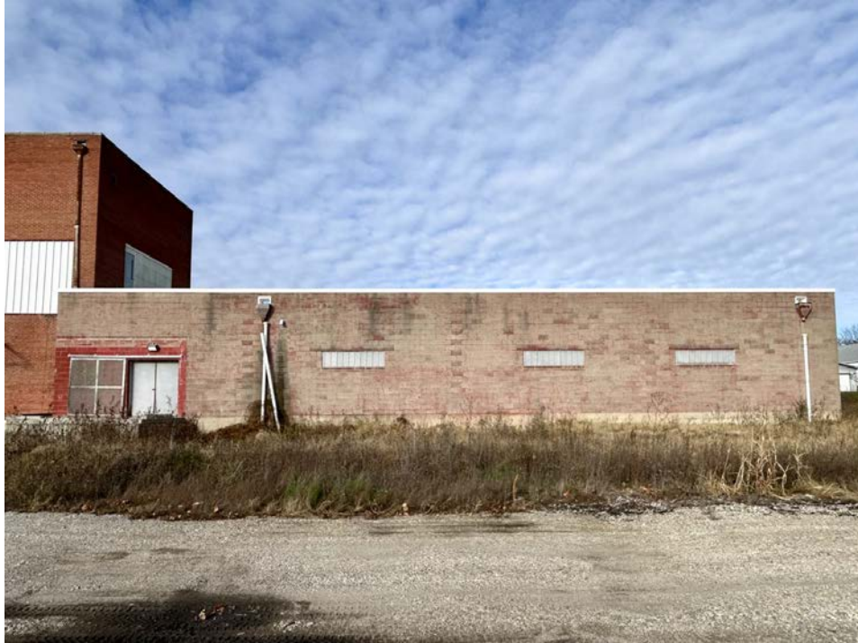
Figure 25: Facing north toward the warehouse at Slack Street and First Street (LS-AS-003-0009, noncontributing).
