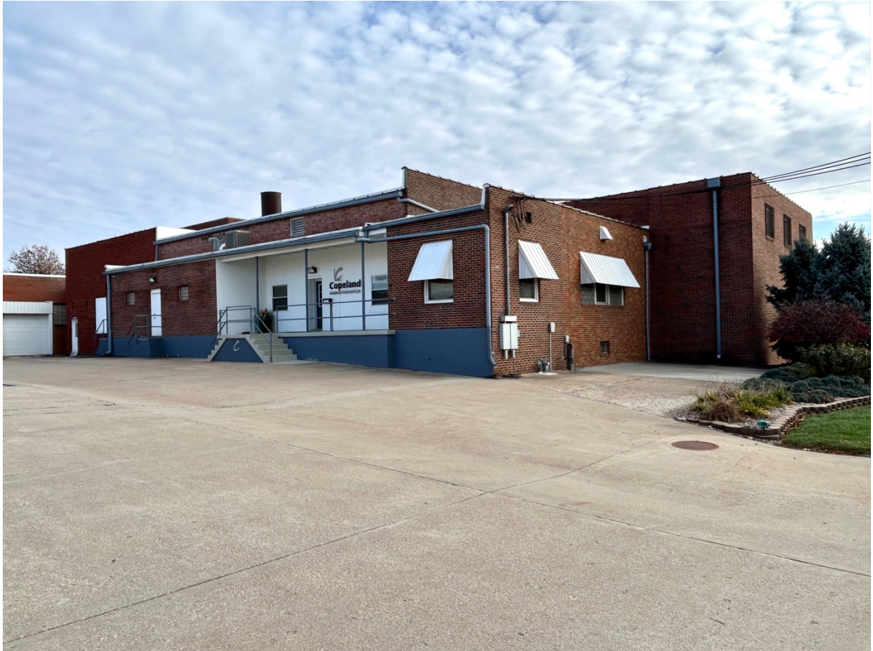
Figure 22: Facing southeast toward the main entrance of the office building of the Producers Creamery complex located at 101 Vine Street (LS-AS-003-0093; Parcel 11-01.00-01-2-17-01.00).
