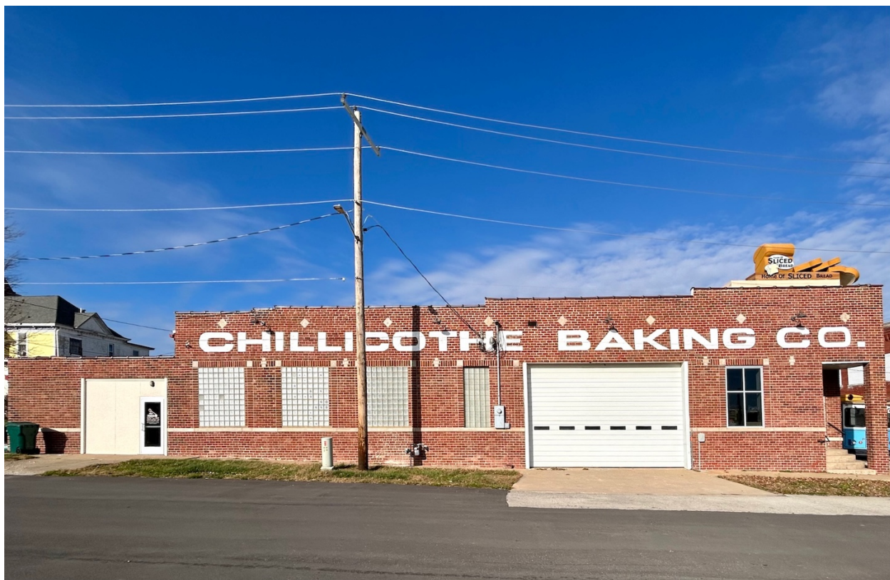
Figure 8: Facing north toward the south elevation of the Chillicothe Baking Company at 100 Elm Street (LS-AS-003-0047; Parcel 11-01.00-01-2-15-05.00).
