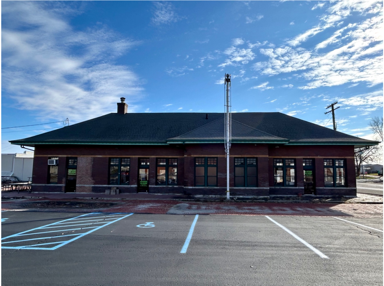
Figure 15: Facing southeast toward the primary northwest elevation of the Burlington & Wabash Railroad Passenger Depot located at 1 Elm Street (LS-AS-003-0046; Parcel 11-01.00-01-2-30-08.00).
