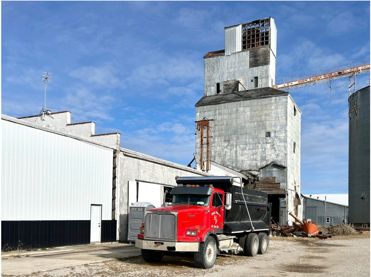
Figure 18: Facing northeast toward the 1953 grain elevator and attached warehouse complex of Milbank Mills located at 1 Henry Street (LS-AS-003-0058; Parcel 11-01.00-01-1-18-01.01).
