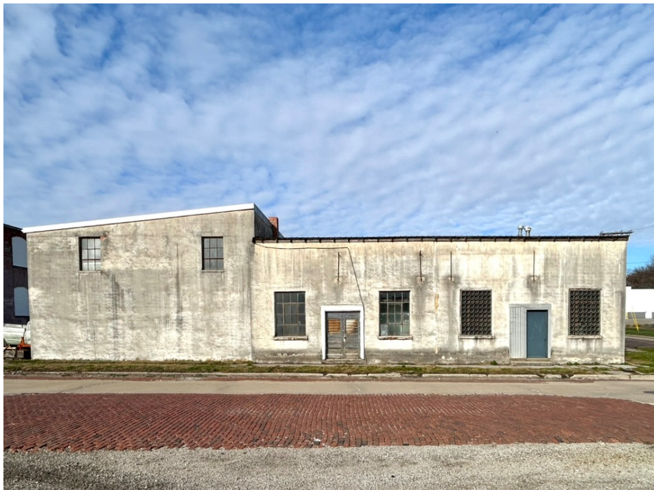
Figure 26: It is recommended as not eligible and noncontributing to the proposed Railroad and Industrial Historic District because of its loss of integrity.
