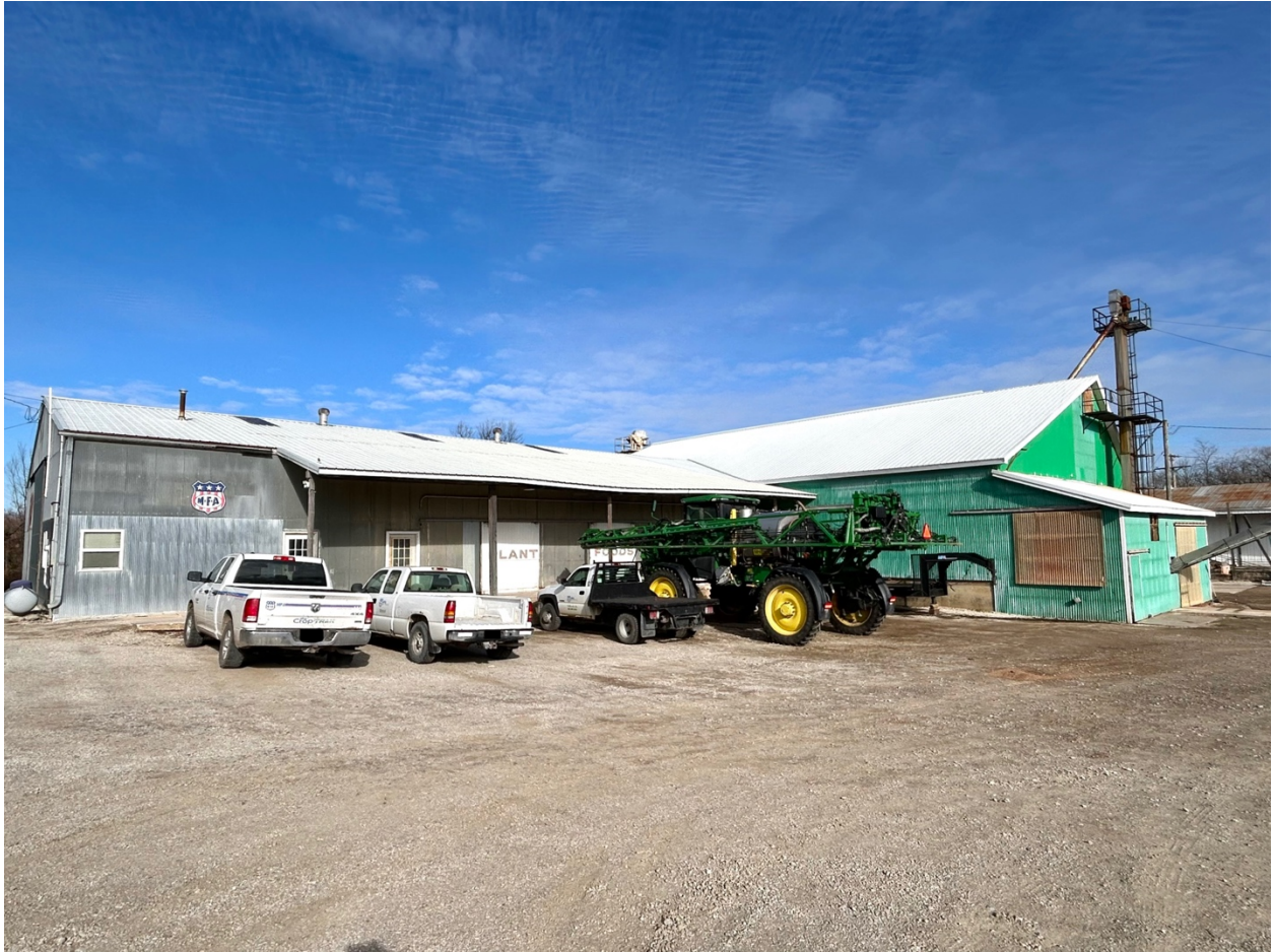
Figure 19: Facing northeast toward the MFA warehouse and fertilizer-storage complex located at 43 Heriford Street (LS-AS-003-0060; Parcel 11-01.00-01-1-18-01.00).
